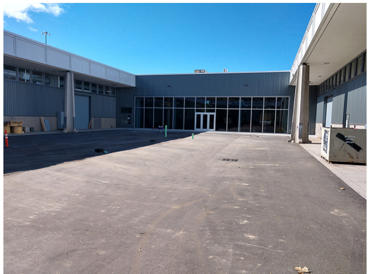
Courtyard area, still under construction
